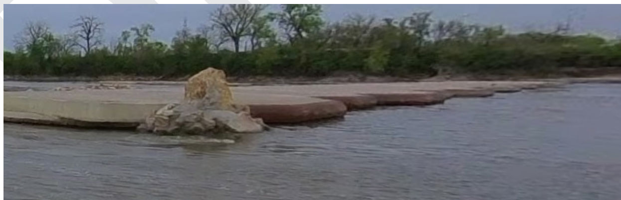
Figure 13. Cellular cofferdam example, on the Kansas River at Topeka (Google Earth)
