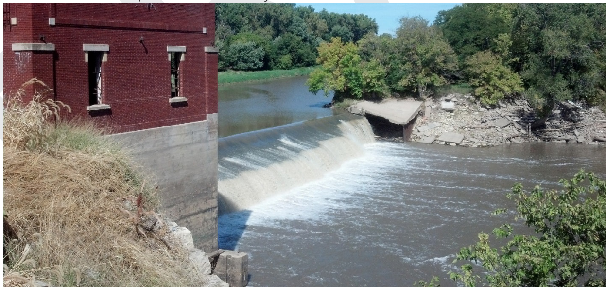
Figure 1. Former Marysville Dam showing hydroelectric plant (foreground)
