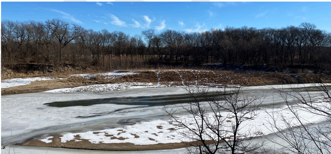
Figure 6. Headcutting just upstream of the failed dam site
